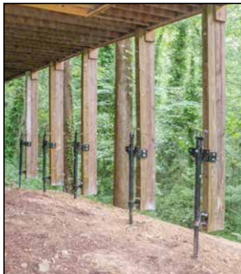
AFTER: Steel piles replaced concrete footings
