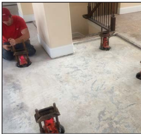
DURING: Installation of helical piles
