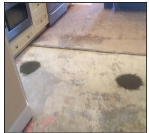
AFTER: Minimal disturbance to interior slab
