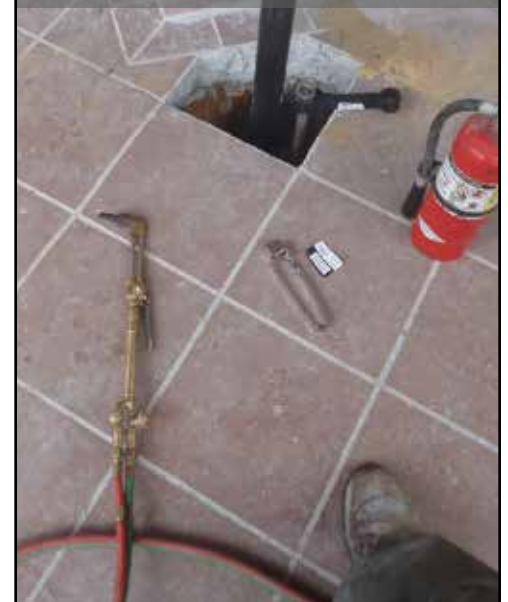
DURING: Minimal removal of concrete during installation
