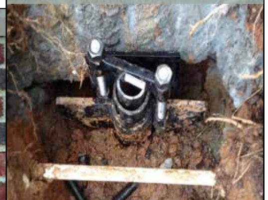
AFTER: 2 7/8 in. piles with standard brackets
