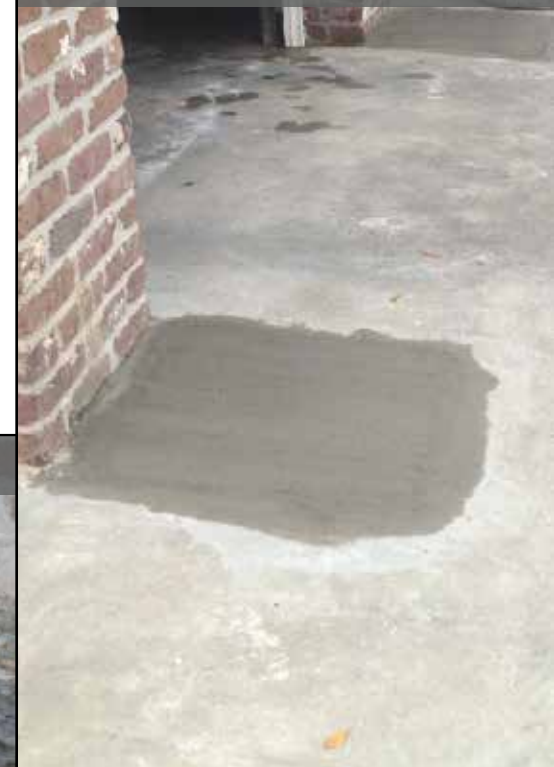
AFTER: Repaired concrete driveway
