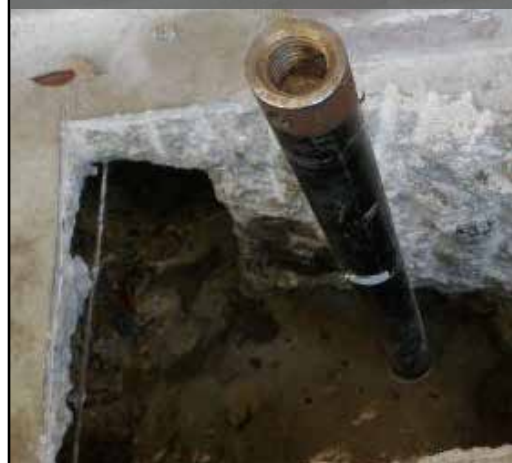
DURING: Helical pile installation
