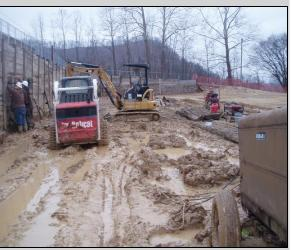
**Solution:** A local engineering firm working with the General Contractor, Solid Rock Construction, specified helicals as a method of repair. We installed seventy-six (76) – 2 7/8" helicals at an average of seventy - (70) feet per pier. Then whalers where installed to support the steel post of the retaining wall.
