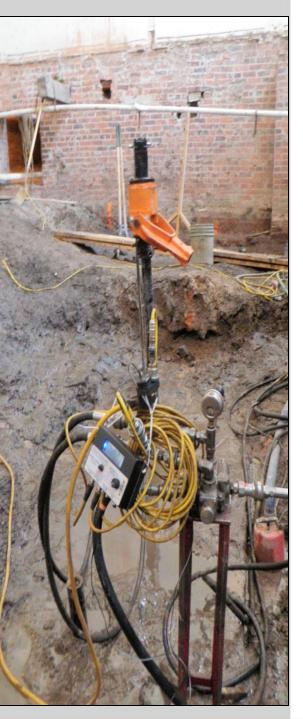
**Conclusion:** The entire project was 167 Ram Jack helical pilings that went 50'- 60' deep. The majority of those were installed manually on the interior (no machine access).
