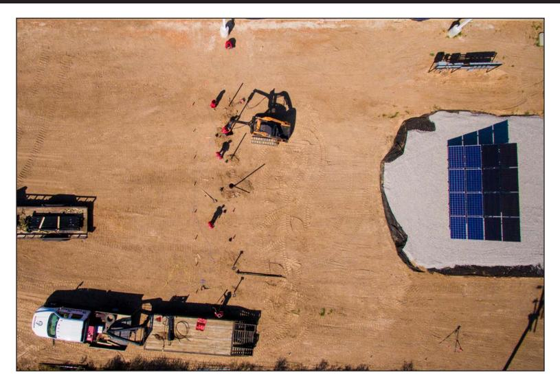
As with any investment in a structure, ensuring the foundations of solar panels can withstand loads is paramount to their longevity. Helical piles have been commonly used as an efficient alternative for ground mount solar panels which are designed with their own support system extending to the ground.
