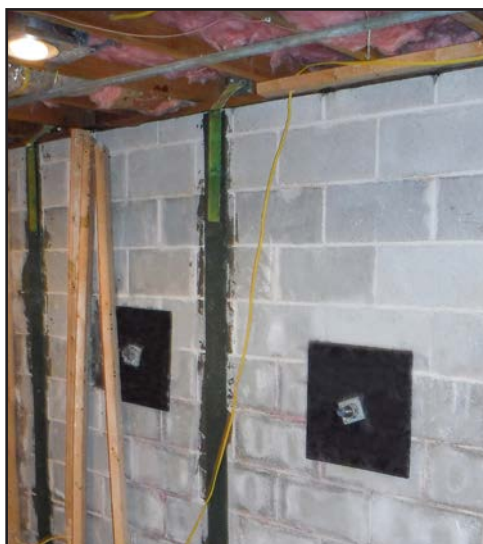
Wall plates shown on the inside of the basement, attached to helical tie-backs
